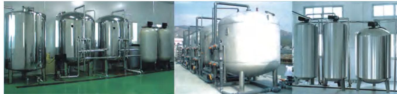
原水箱、机械过滤器、活性炭吸附器、软化器 Water tank, mechanical filter, active carbon absorber, softener
